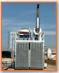
In a cogeneration system, endothermic machines are used to generate both electricity and heat from a single primary energy source, for instance a combustible gas such as natural gas, bio-gas, landfill gas, flare gas, etc.
