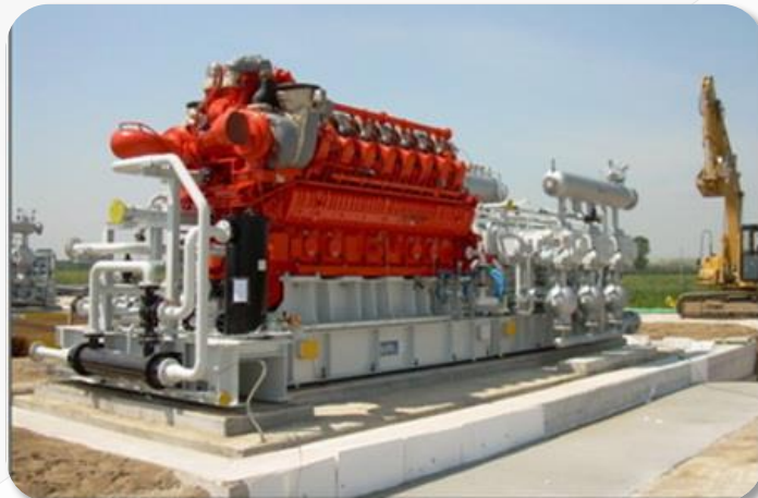
BORDOLANO ITALY – UNDERGROUND STORAGE
