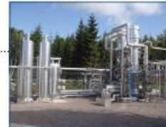
Pressure and Temperature Swing Adsorption System
