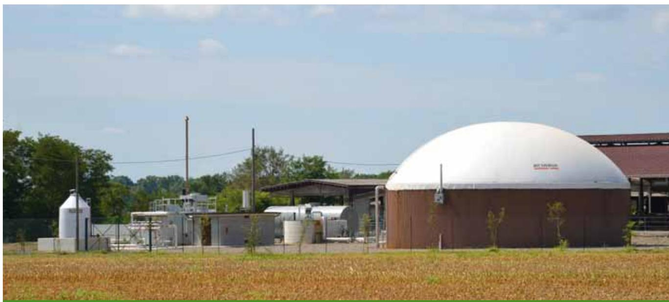
*Impianto 100% liquame e letame bovino da 100 kWe - 100 kWe biogas plant with 100% cattle sewage and manure*
