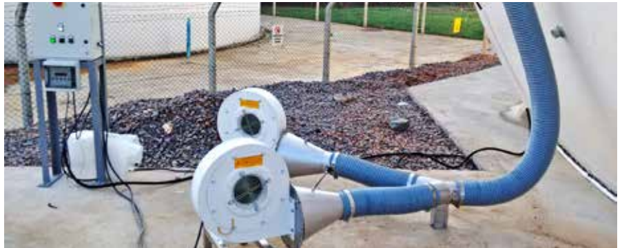
CENTRIFUGAL AIR FANS WITH ELECTRICAL PANEL
