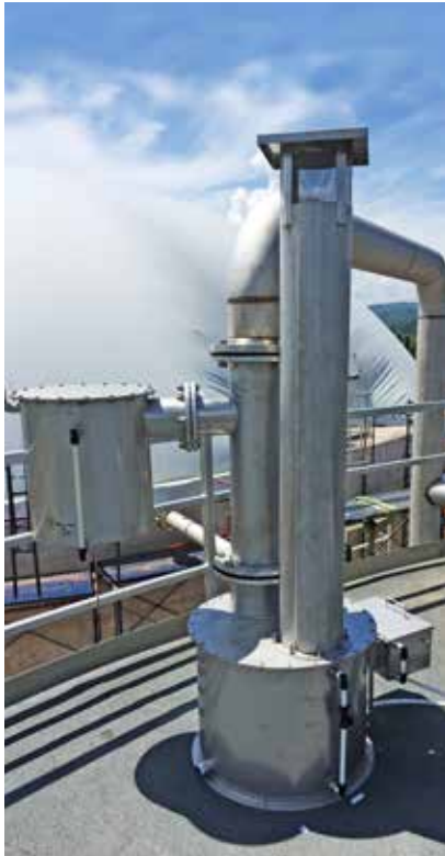
HYDRAULIC SAFETY VALVE WITH ANTI-VACUUM
