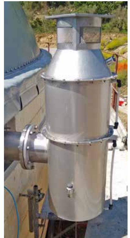
OVERPRESSURE AND ANTI-VACUUM SAFETY VALVE
