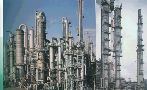
Chemical Plant (EG & NH 3 )
