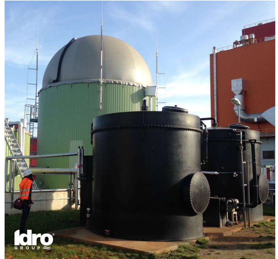
Biogas desulphurization from anaerobic digestion percolate waste from an incineration plant Zona Erfurt - Gera
